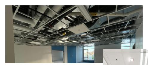
The School is using ACT Ceiling Panels that are used to reduce noise by absorbing sound waves and minimize reverberation.
